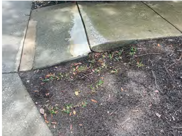
Image 14 Grinding lifted sidewalk sale is only a temporary fix. The slab will be refitted by the roots within months or a year or two.
