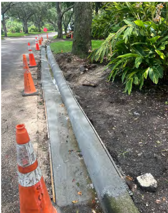
Image 15 This curb repair photo was taken on June 2, 2025. At least one large 9-inch diaper root was cut within 12 inches of the tree. This destabilizes the tree.
