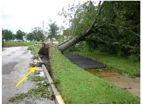
Image 7 When root growth is restricted by infrastructure, the roots cannot anchor the tree properly making it more likely to fall over in a wind event. Roots can often eventually break out of the restrictions by damaging the infrastructure. Above one root grew under the curb causing the curb to come out when the tree fell. (Yellow arrow) (Photo by author taken at another site in St. Augustine after Hurricane Francis in 2004.)
