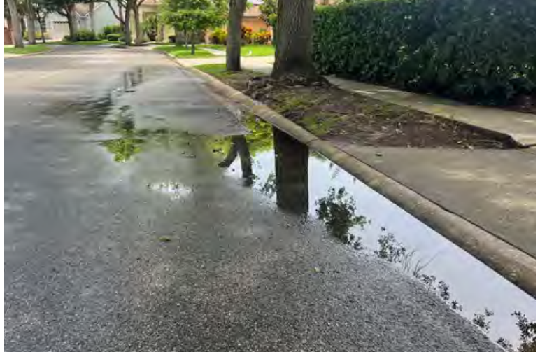
Image 5 The roots of this tree have raised the curb and gutter and the nearby asphalt breaking the drainage flow resulting in long-term damage to the road subbase and expensive future repairs.
